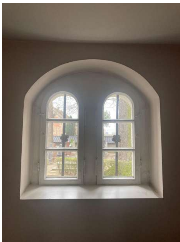
Fot. 43. Stolarka okienna, widok wew.
